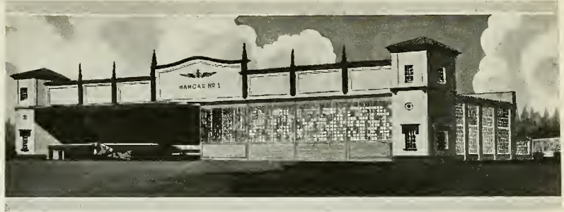
One of the two cantilever hangars included in the initial construction project
